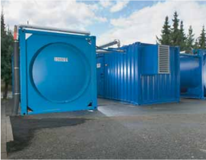
90 kW vegetable oil powered CHP unit in a container with 25 m 3 main tank and buffer tank.
